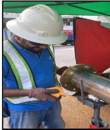
Pipe measurement work
